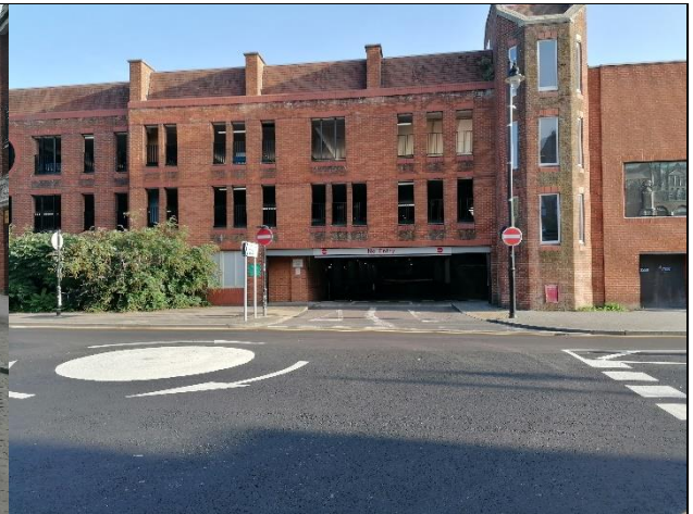
Photograph 2: Kennet Centre MSCP Exit
