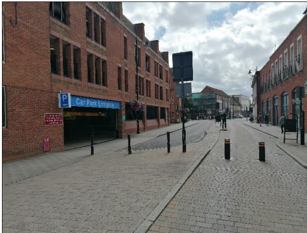
Photograph 1: Kennet Centre MSCP Access
