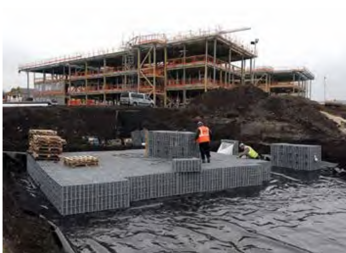
Figure 21.1 Geocellular storage system under construction (courtesy Polypipe Limited)
