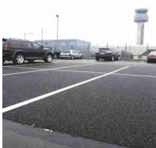
Figure 20.3 Car park at East Midlands Airport with porous asphalt surfacing (courtesy EPG Limited)
