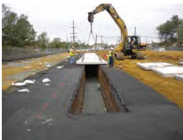
Figure 21.15 Hybrid tank of reinforced earth and concrete roof panels (courtesy Stormwater Management)
