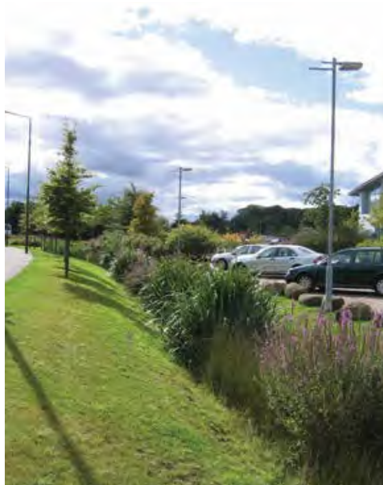
Figure 17.11 Linear wet swale, Junction 4 M8, West Lothian
