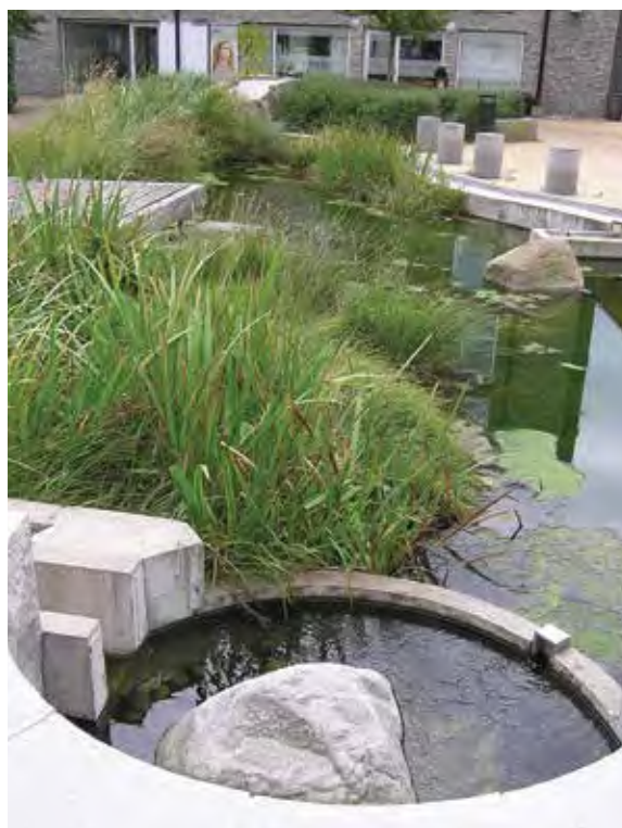
Figure 23.7 Pond with baffles and islands, Augustenborg, Sweden
