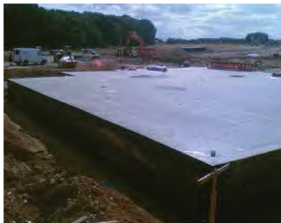
Figure 21.3 Frame covered by outer skin (geomembrane in this case) (courtesy EPG Limited)
