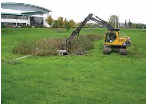
Figure 32.2 De-silting (courtesy Bedford Group of Drainage Boards)
