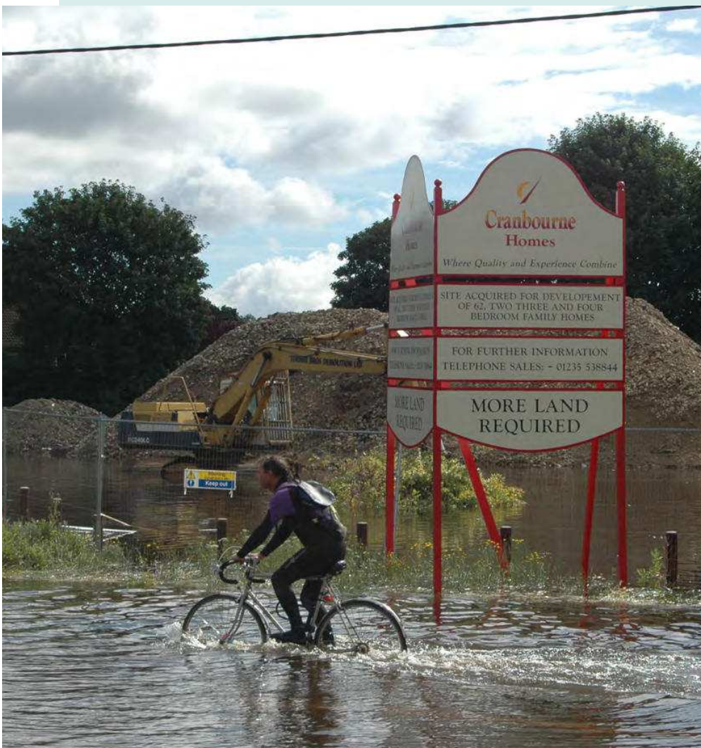
Flooded development site (© JBA Consulting)
